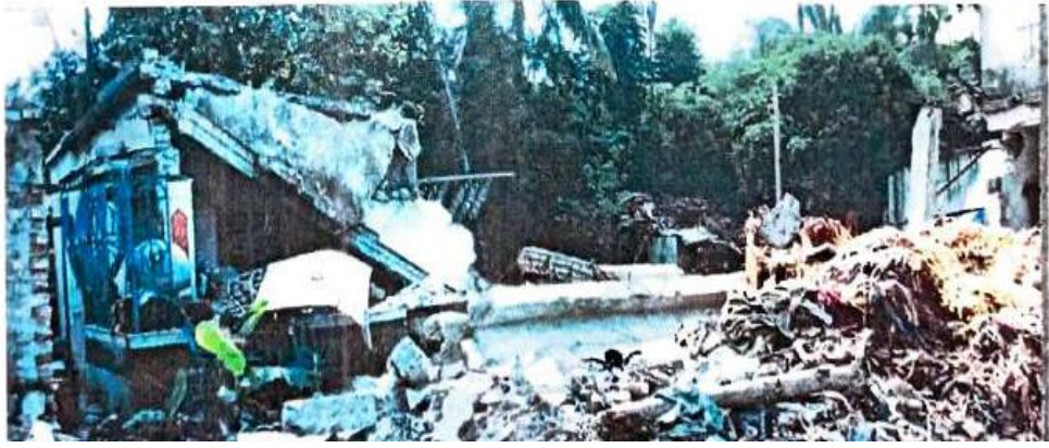
Fig.2 Damage of adjacent nearest Household/Building due to blast (photo taken on 10.10.2023)
