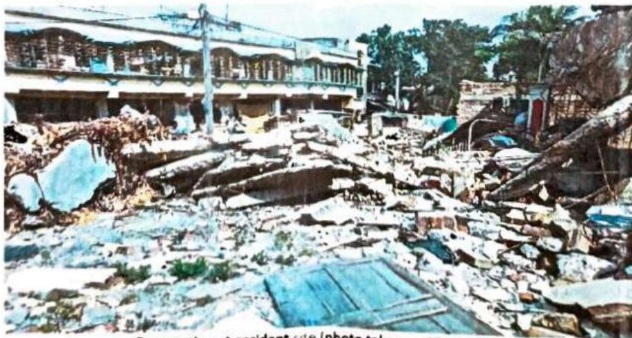
Devastation at accident site (photo taken on 10.10.2023)
