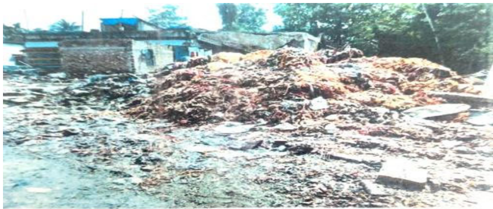
Fig. 1. Alleged Site where incident occurred (photo taken on 10.10.2023)
