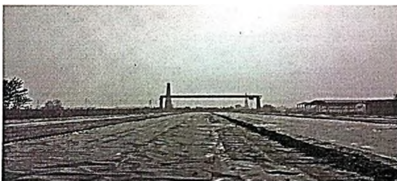
RMS Area with Overhead Crane Actual Image
